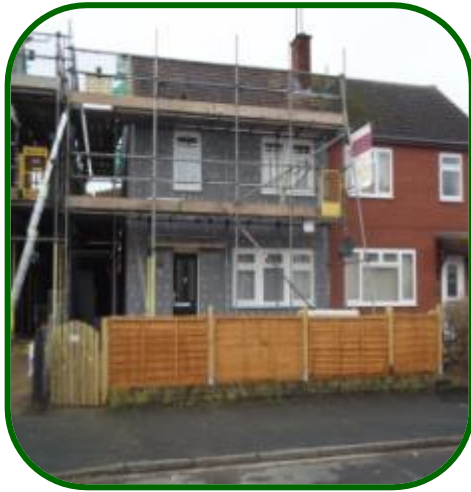
External Wall Insulation in Hucclecote
