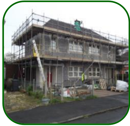
External Wall Insulation in Hucclecote
